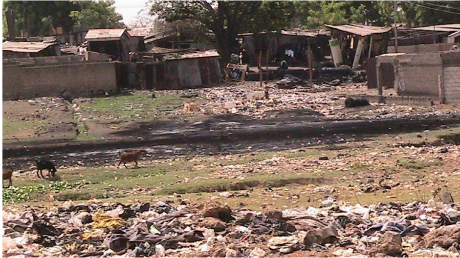
Fig. 3: Another view of waste dumping at the lake site
